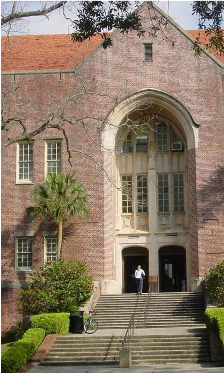
Photo 15.15 Building Raised on Small Podium
