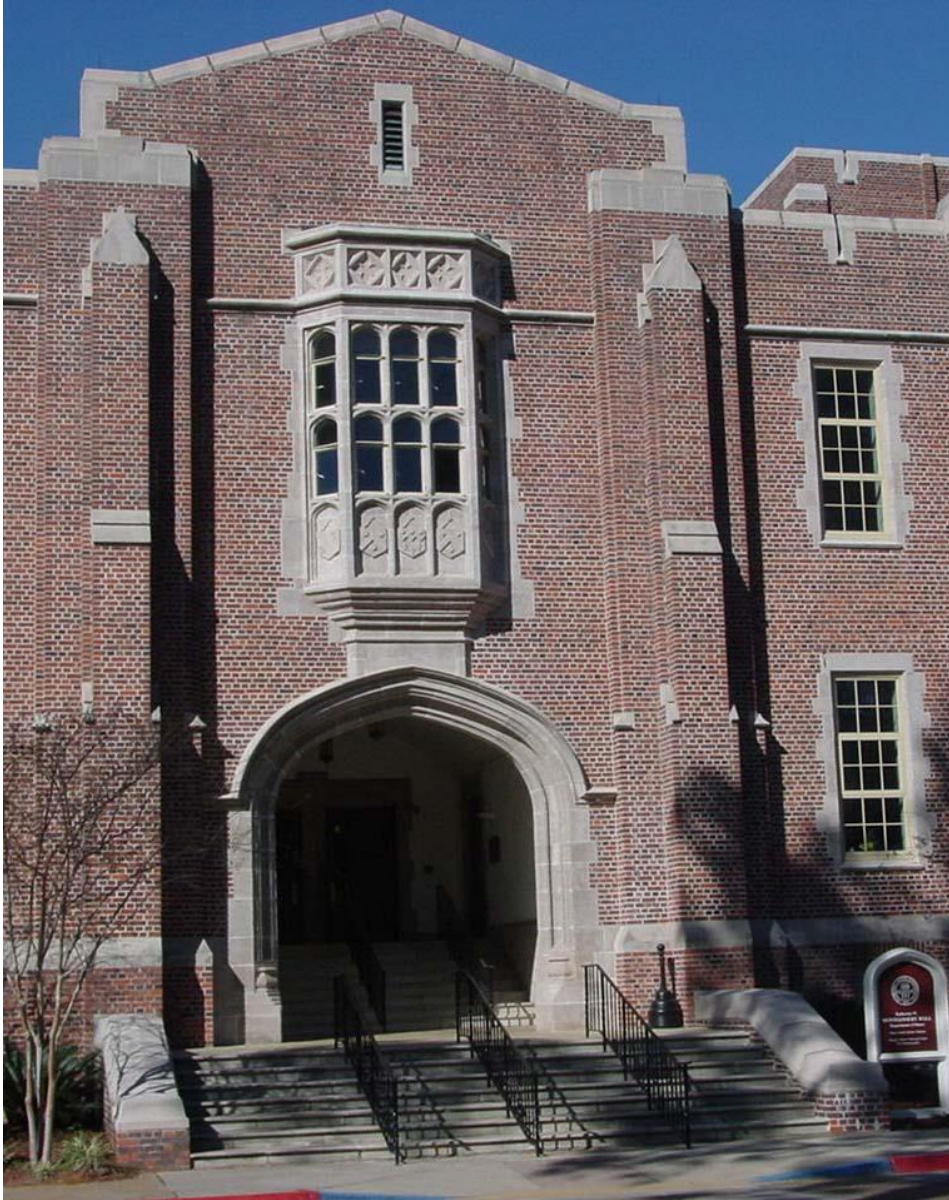
Photo 15.6 Jacobean Arch and Proper Gable/Pier Design (Montgomery Gymnasium)
